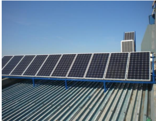
Figure 1. Fixed on-grid 2 kW p PV system in Niš, Serbia
